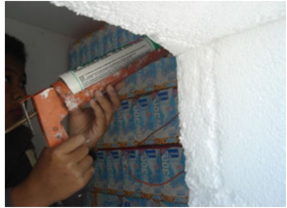
Figure 4. The tested wall was installed with the panel of used milk containers filled with rice husk.
