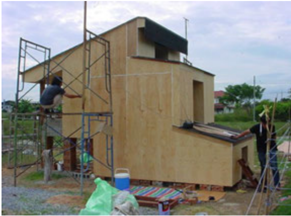
Figure 2. The physical character of simulated building that installed with the insulation from rice husk at its external wall.
